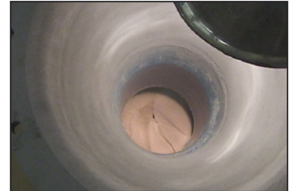
Ash cone after molding ARC MX1 in place
